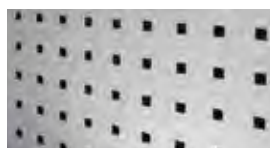
perforirane stene, luknje dimenzije 10 x 10 mm, raster 38 mm
